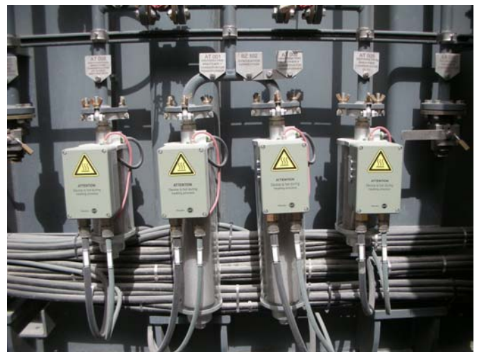
Fig. 2 MTrab, maintenance free breather
